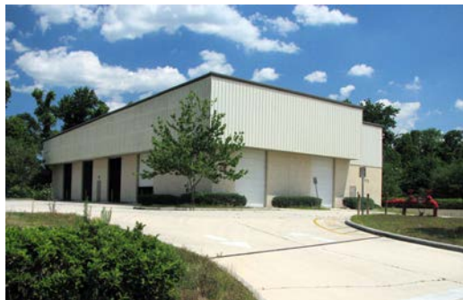
General use Multi-tenant Industrial/ Distribution Warehouse
