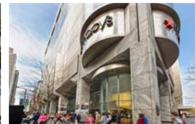
Water Tower Place, Chicago, IL
