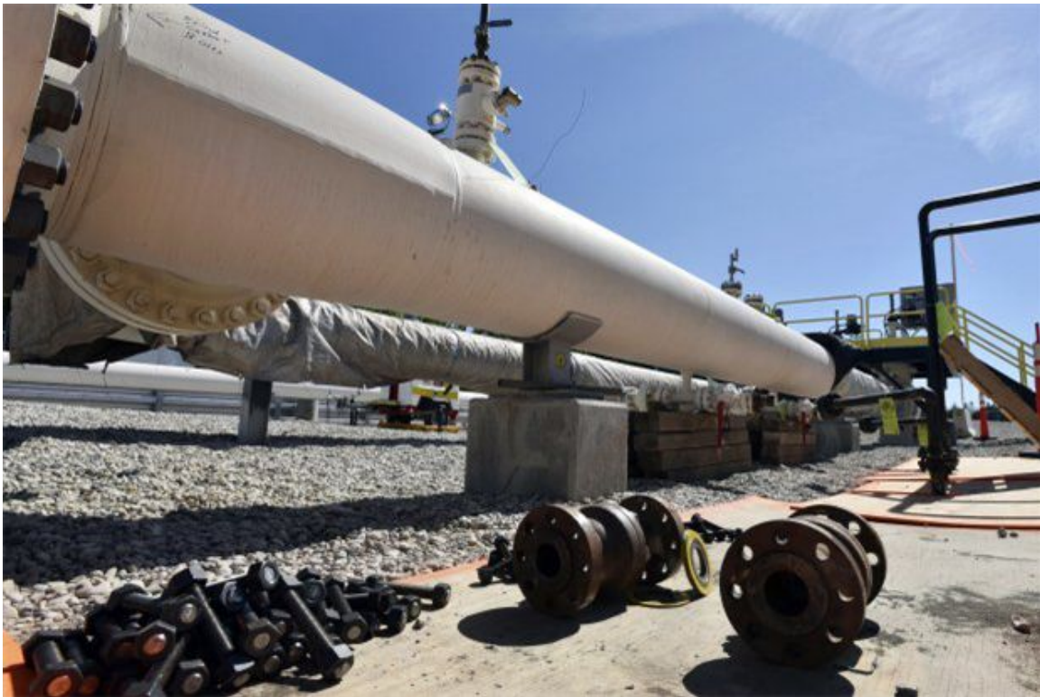
A pipeline near St. Ignace, Mich. PHOTO: DALE G. YOUNG/ASSOCIATED PRESS
